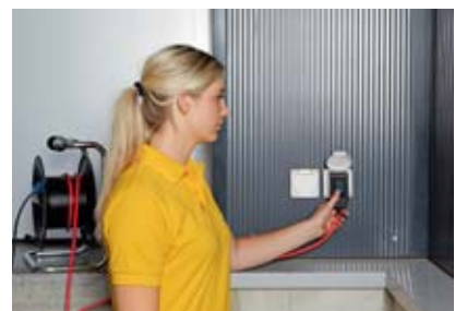
3 Mobiler FI-Schutz (RCD)
